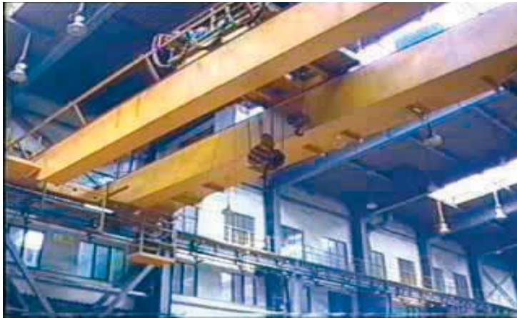
Rys. 5. Obiekt bada - suwnica pomostowa Fig. 5. The object investigates - the bridge-gantry
